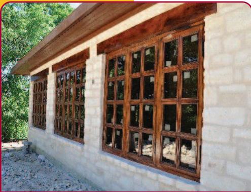
THE NORTH END OF THE LODGE IS NOW COMPLETE.
